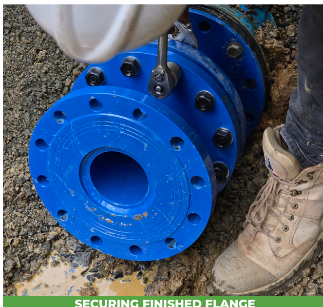
SECURING FINISHED FLANGE
