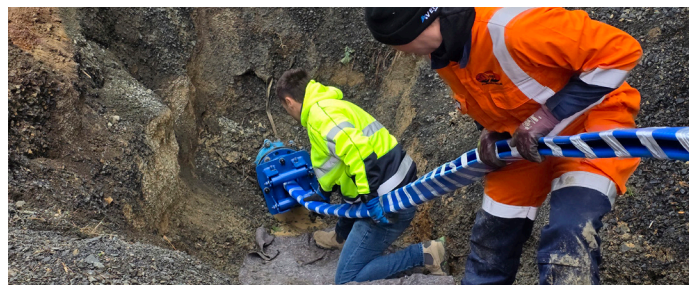
PULLING LINER INTO PLACE
