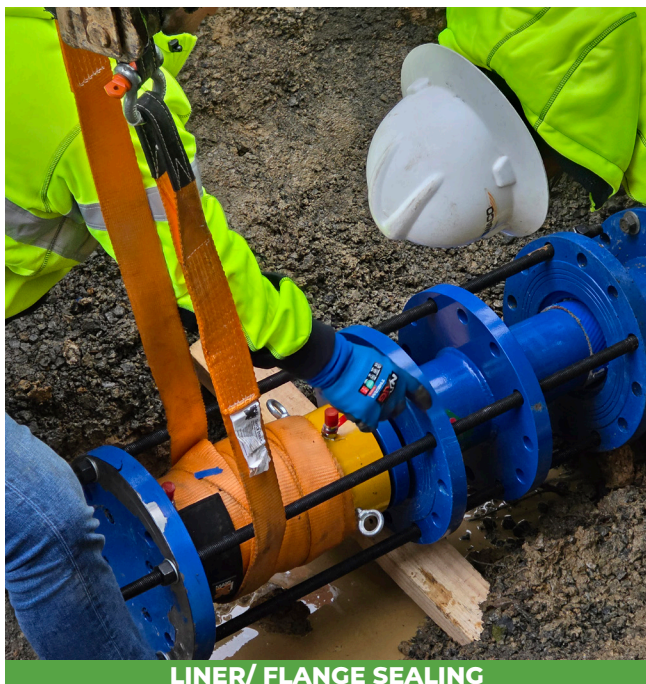
LINER/ FLANGE SEALING
