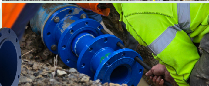
SECONDARY FLANGE INSTALLATION
